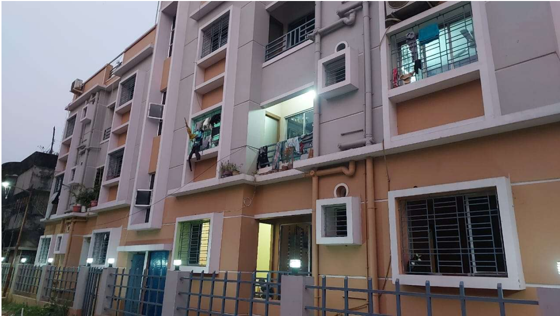
vii) front view of Building
